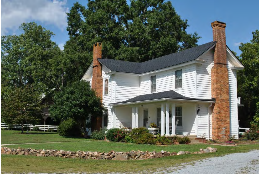
James Newton Plaster House, Façade, Looking East.
