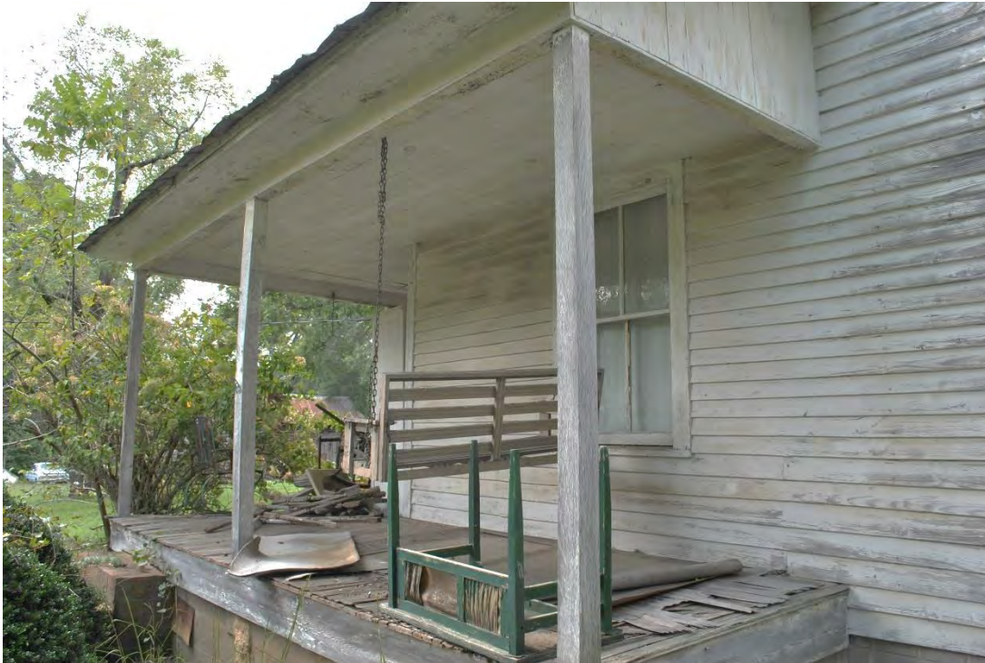
Blackwelder Family House, Front Ell, Porch Along East Elevation, Looking Southwest.
