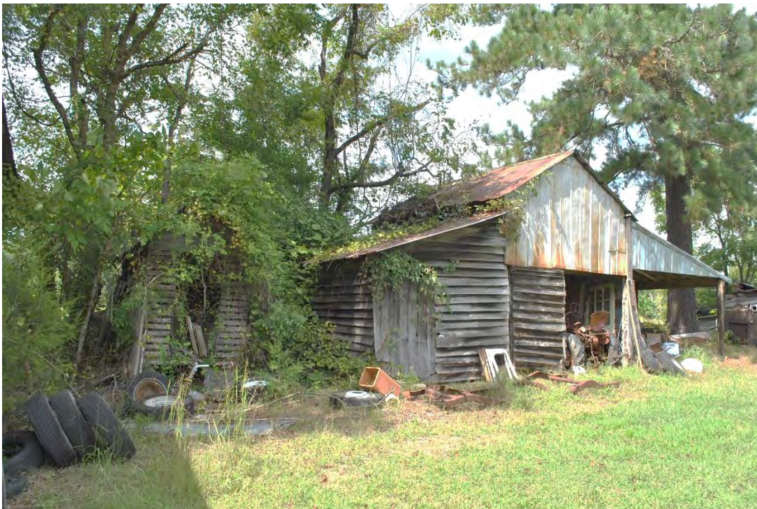
Blackwelder Family House, Corncribs, Looking West.
