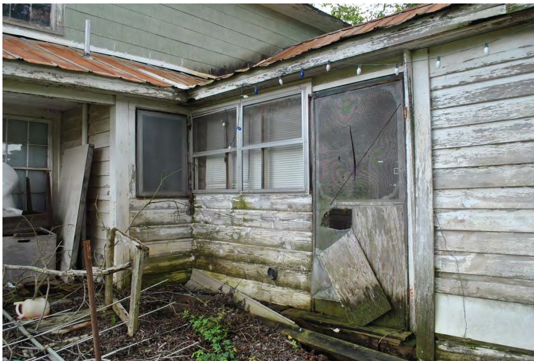
Blackwelder Family House, Rear Ell Porch, Looking Southeast.
