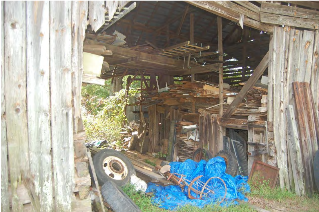
Blackwelder Family House, Log Barn, Center Passage, Looking South.
