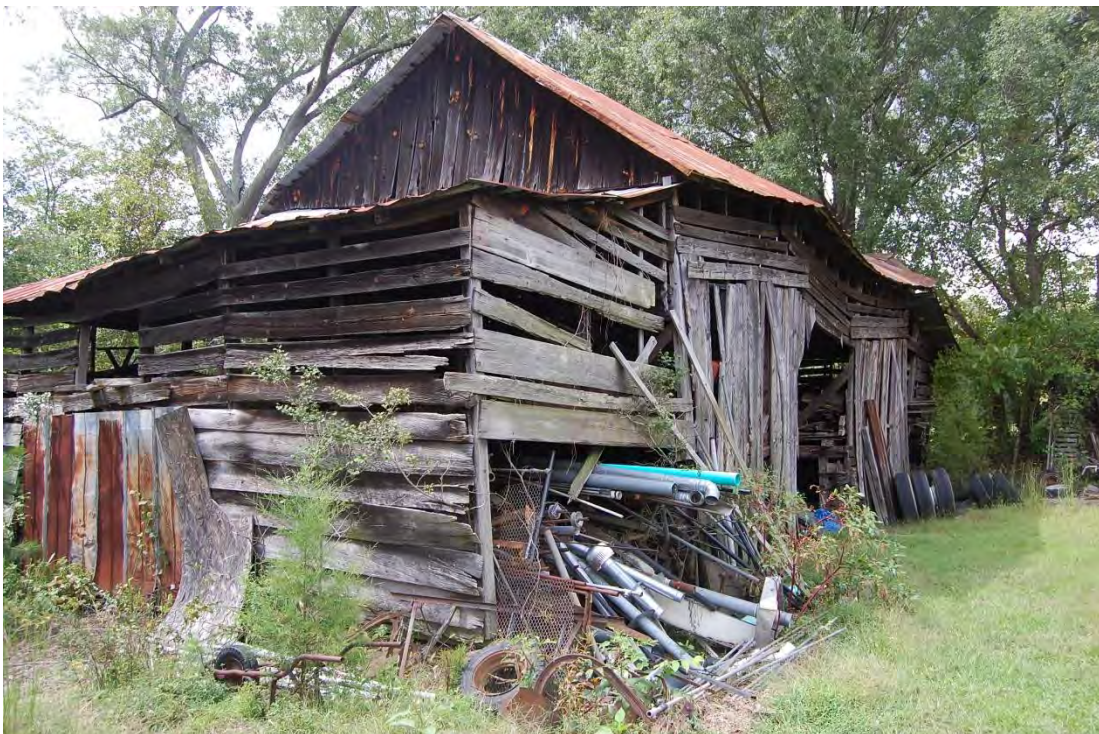
Blackwelder Family House, Log Barn, Looking West.
